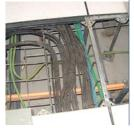
VESDA sampling pipe should be installed under the restricted area of the raised floor and near high-risk cabling, this enables early detection of any smoke in that space.
